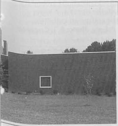
ty College in Hamlet was lege library, a guided studies he LRC. y Architects, (Wilmington, NC) Photo: Chuck Lowery
