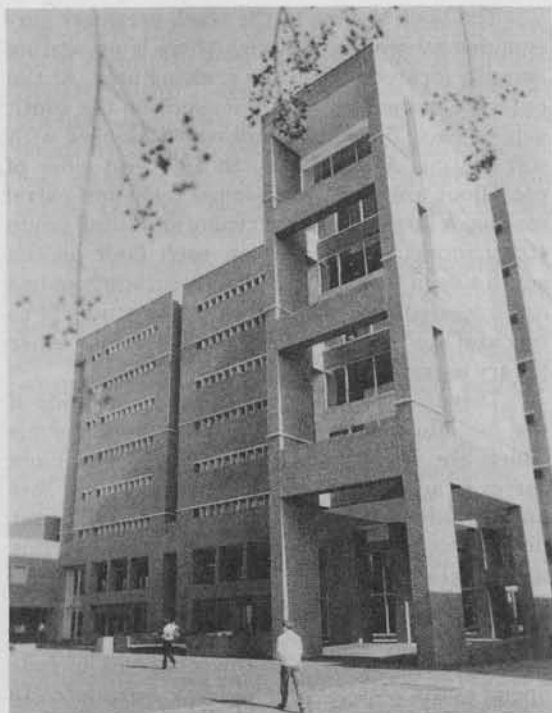
A view of the west end of the Davis Library. The entrance to the building is located at the far left under the arcade. (Photo by Will Owens, UNC News Bureau.)
